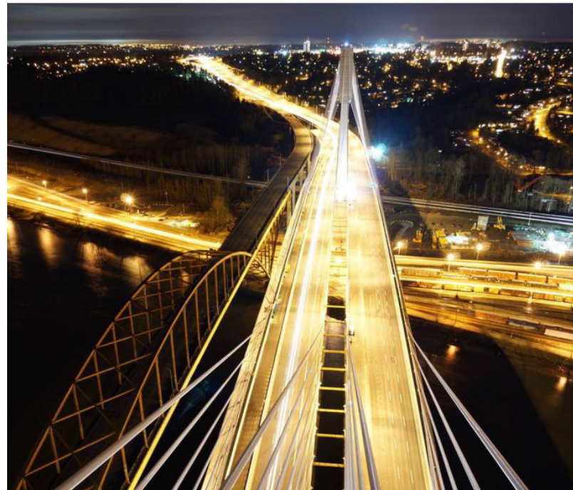
Two decades after going open shop, Kiewit built the spectacular Port Mann Bridge
